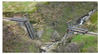
Far below you on the right, you will see a water catchment system. Water from the Furkareuss is guided through an 8 km long tunnel to the Göscheneralp reservoir, and then on to the Swiss Federal Railway's hydroelectric power stations at Göschenen, Wassen and Amsteg.
